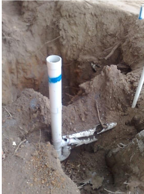
Trench failures occur due to incorrect installation and poor compaction.
