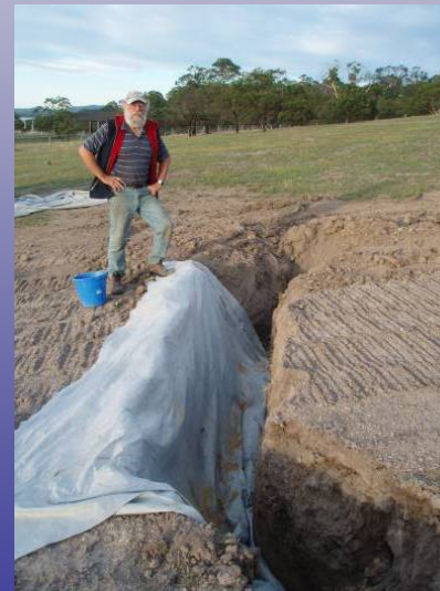
Fill with fine sand and gypsum 5% wt
