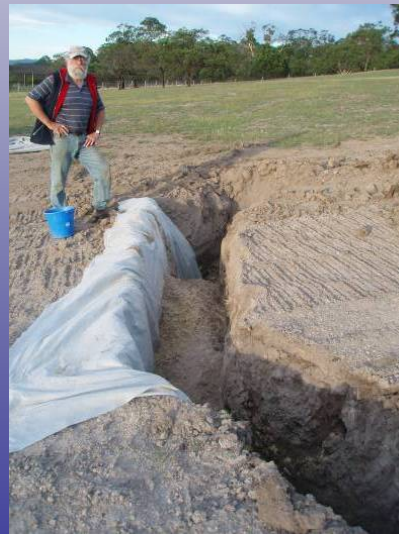
Geotextile downslope wall
